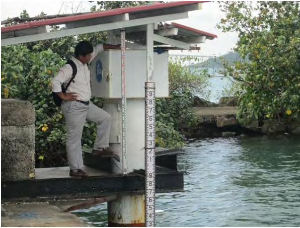
Leveling survey from PAS BM point to Tide Station BM point
