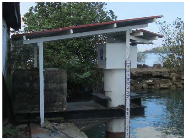
The close-up view of Tide Station.
