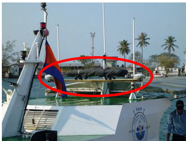
GNSS Antennas Installation
