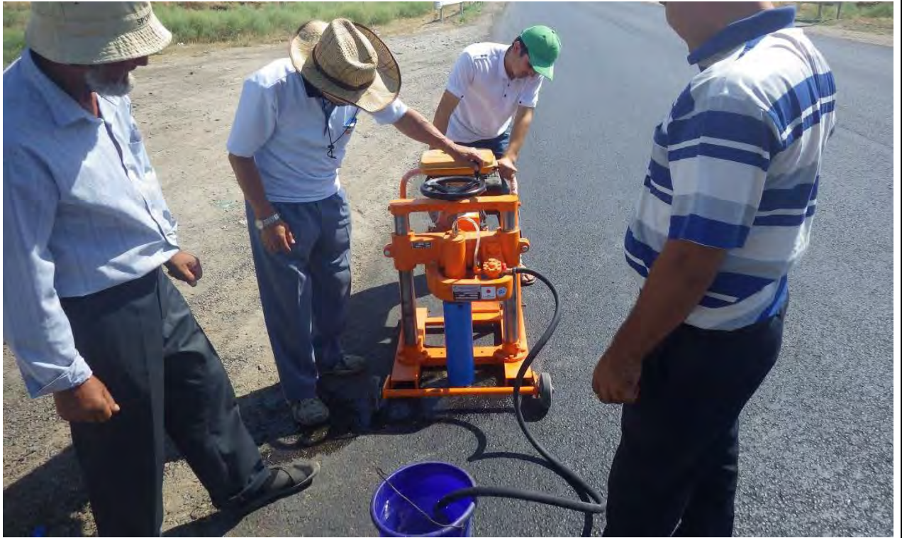
Installation of JICA supplied laboratory equipment Figure7
