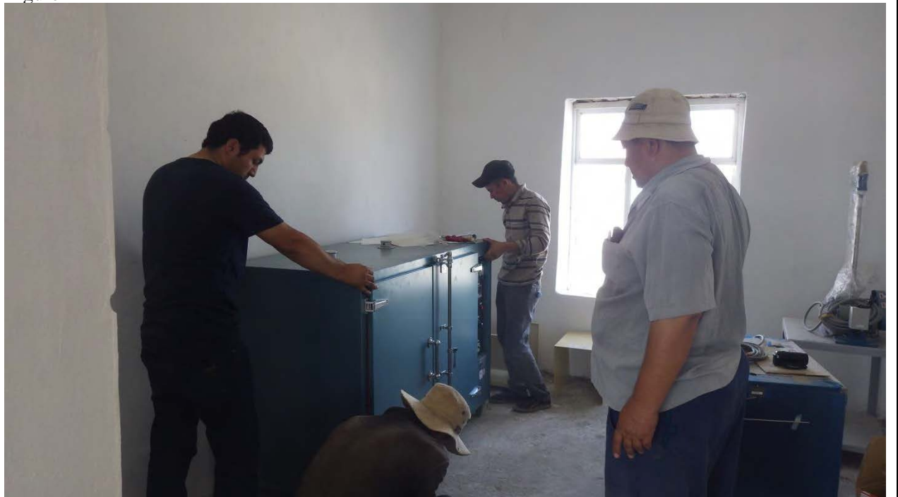
Installation of JICA supplied laboratory equipment Figure 2
