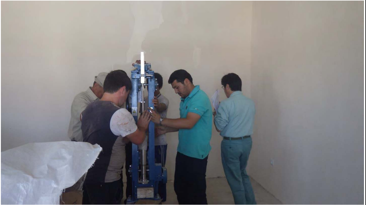
Installation of JICA Supplied Laboratory Equipment Figure 1
