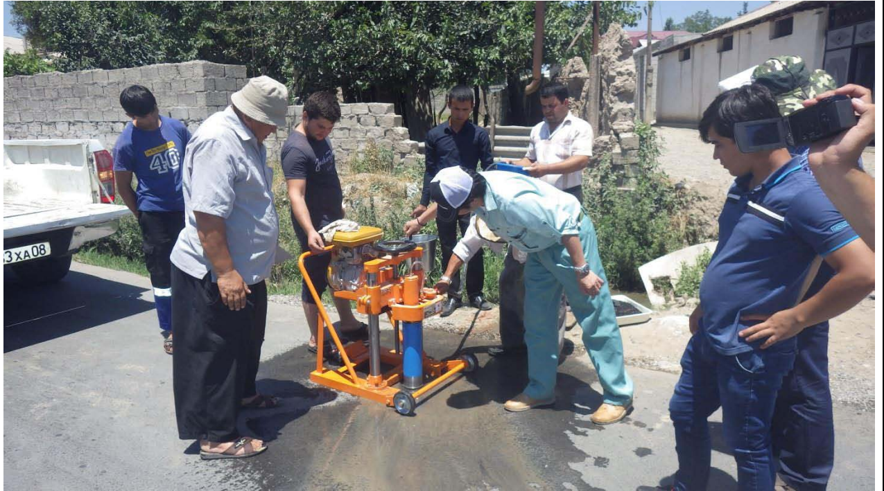
Installation of JICA supplied laboratory equipment Figure7
