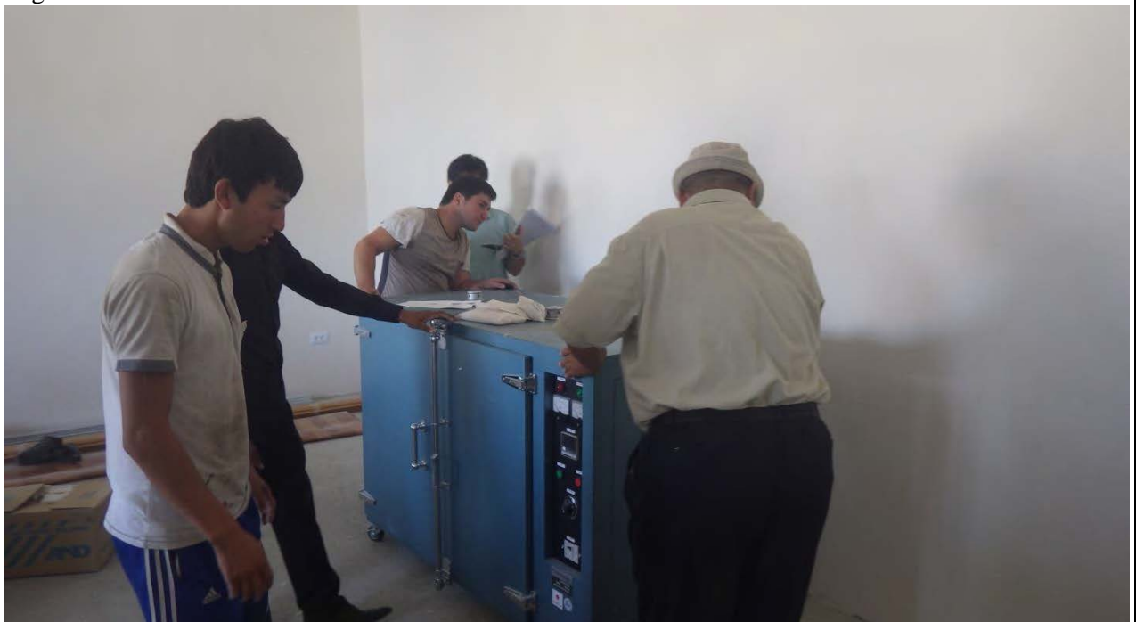
Installation of JICA supplied laboratory equipment Figure 2
