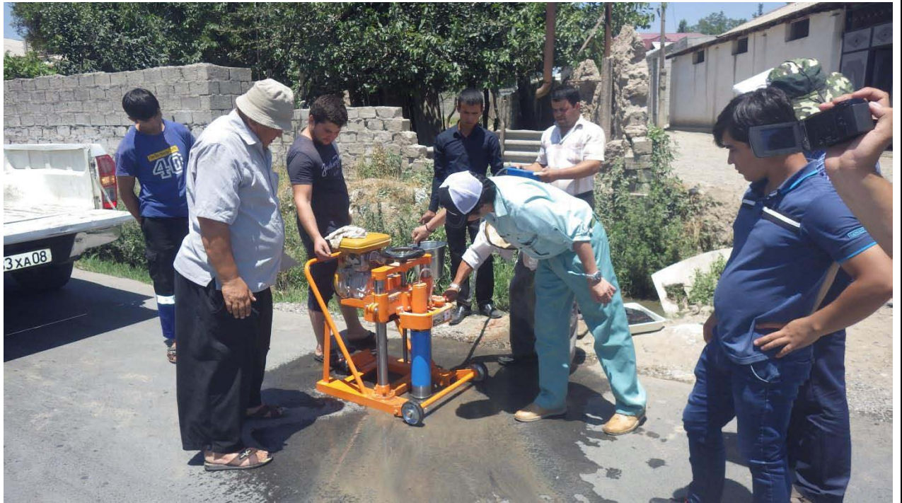
Installation of JICA supplied laboratory equipment Figure7
