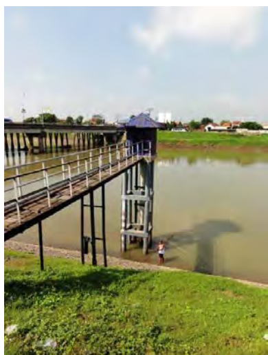
Porong water level gauging station
