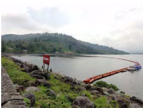
Screen for intake at Selorejo Dam
