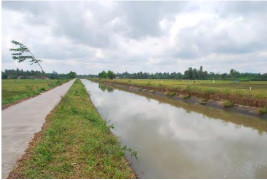
Photo B-1-5: Irrigation channel for the Komerung irrigation system.
