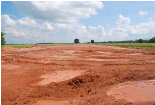
Photo B-1-7: Extension project of an irrigation channel of the Komerung irrigation system to Lemping district.
