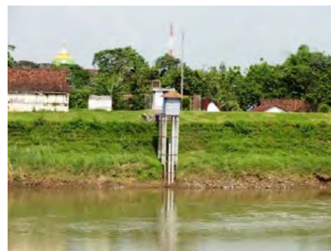
Ploso water level gauging station
