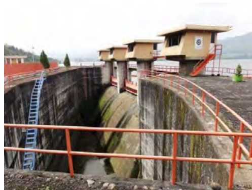
Spillway at Selorejo Dam
