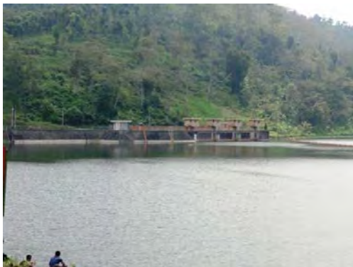
Reservoir at Selorejo Dam
