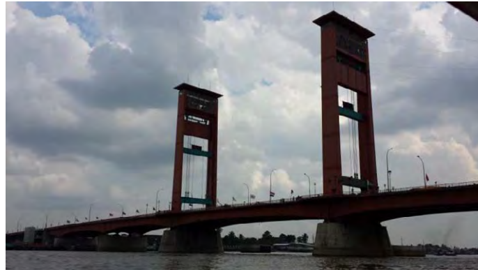
Figure 4.3.1-1 Downstream of Musi: Ampera Bridge, Palembang, South Sumatra.
