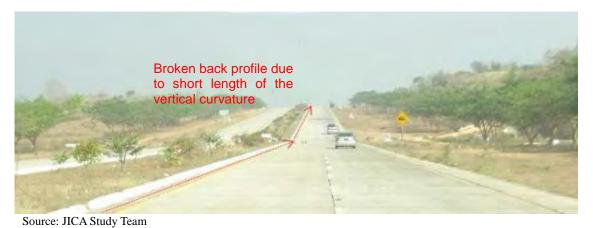
Figure 6.2.14 Lack of Length of Vertical Curvature
