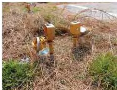
(Damaged Aviation Lights)
