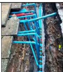
Photo-81 Connections by each customer
