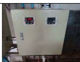
Photo-9 Equipmtent for setting frequency
