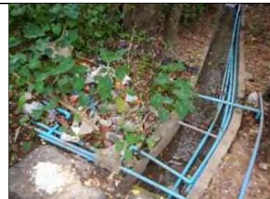
Photo-63 Service pipes above ground
