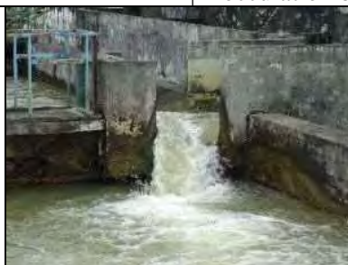
Photo-14 Outlet of flocculation basin in the Phase 1
