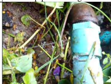
Photo-65 Leakage on service equipment
