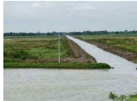
Photo-1 Raw water conveyance channel (Open channel)
