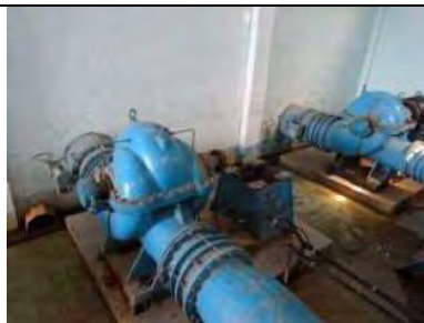
Photo-3 Intake pump without electric motor
