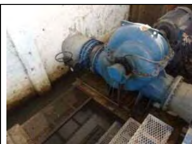
Photo-5 Leakage through gland packing
