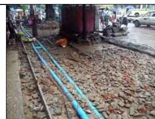
Photo-72 Laying distribution pipes
