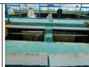
Photo-10 Coagulant injection point
