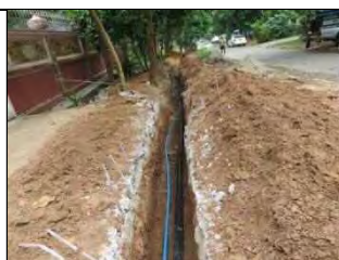
Photo-71 Laying distribution pipes
