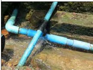
Photo-64 Leakage on service pipe
