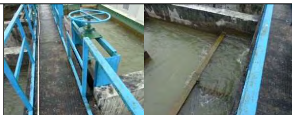
Photo-12 Large opening of inlet gate of flocculation basin
