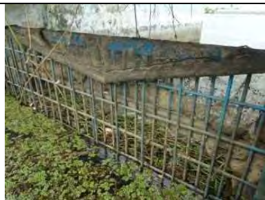
Photo-2 Inlet gate of intake pump well, Front: Pump well Back: Pre-sedimentation basin,
