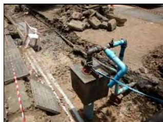
Photo-67 Connection with tube well water
