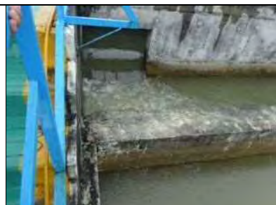
Photo-15 Outlet of flocculation basin in the Phase 2
