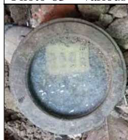
Photo-84 Impossible to read meter data
