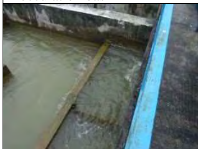
Photo-13 Over flow on the wall of vertical baffled channel
