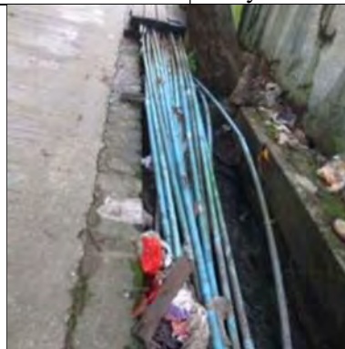
Photo-62 Service pipes above ground
