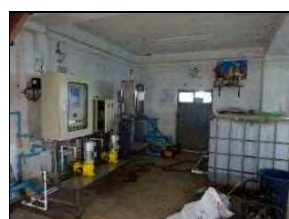
Photo-7 Cogulant injection facilities
