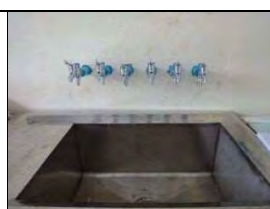
Photo-45 Taps for collecting water sample
