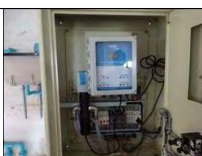
Photo-8 Broken turbidity meter
