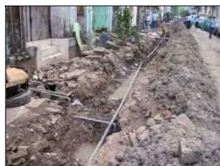
Photo-70 Laying distribution pipes
