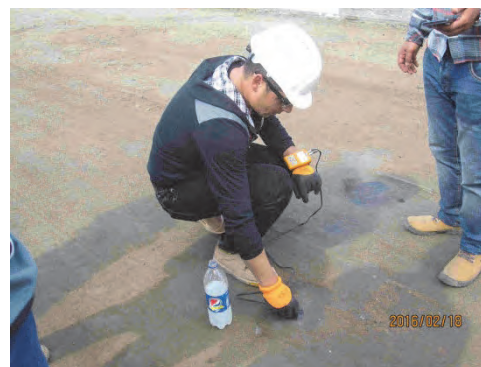
2. Measurement of Steel Deck plate
