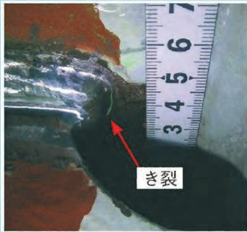
Removal of cracks by grinding.
