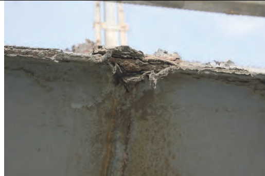
Severe corrosion
