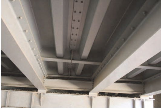
11. U-ribs and adjacent U-ribs directly above the longitudinal beam and consisting of two inclined plates.
