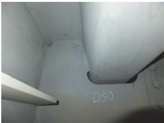
5. D50 diaphragm, east face. No cracks.
