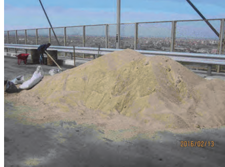
2. Sand for sand blasting
