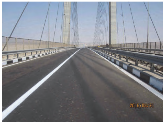
The surface of pavement of North Side.
