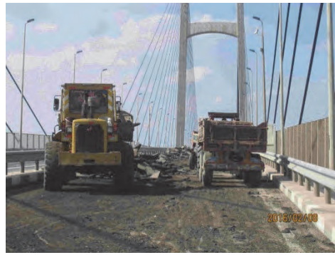
2. Taking away removed asphalt.
