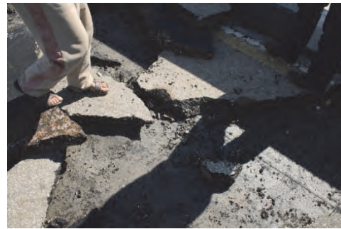
6. Steel deck near center median. No rust is seen here.
