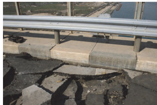
6. P13, Removed pavement and a cap on pavement.
