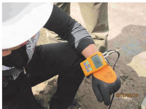
1. Measurement of Steel Deck plate
