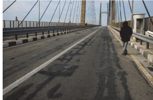
2. Driving Lane and 5 lines of pavement repair are visible. These lines correspond to the center of the U-ribs or the center of two adjacent U-ribs.
