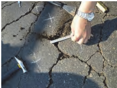
Photo1.2.1 Detailed Inspection for damaged pavement
