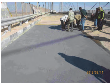
5. After sand blasting
