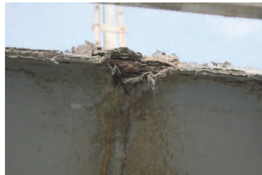
10. Severe corrosion
