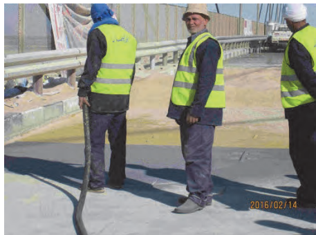
1. Work of sand blasting
