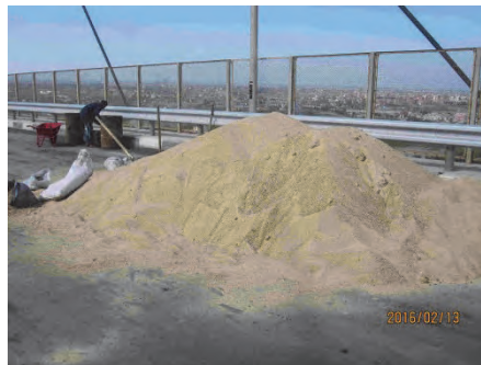
2. Sand for sand blasting
