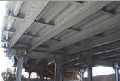
2 The structure of the orthotropic steel deck panel adopted for the Maasara Bridge resembles the structure of the orthotropic steel deck adopted for the Suez Bridge.
