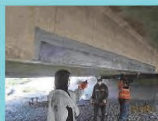
Final coating of Epoxy adhesive
