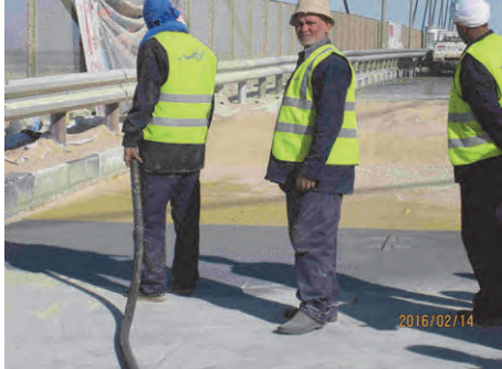
1. Work of sand blasting
