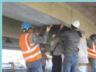
Setting of CF (Carbon-fiber)
