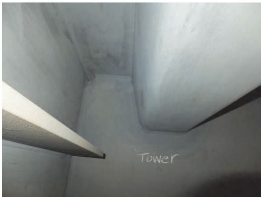
3. Only south side R8 U-rib is shown. D30, East face at Tower. No paint cracks were found.
