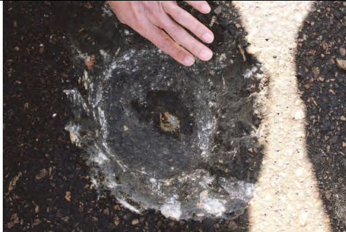
3. Condition of pavement was quite good and no rust was observed on the deck surface. The yellow color shows the Zinc Chromate.
