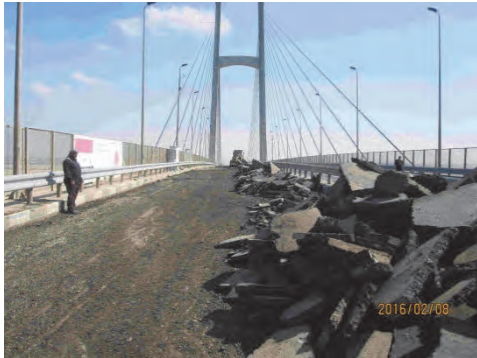
1. Removal of pavement on east side.
