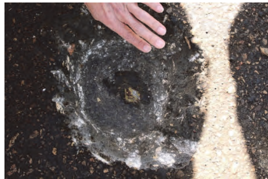
4. Condition of pavement was quite good and no rust was observed on the deck surface. The yellow color shows the Zinc Chromate. Hexavalent(+6) Chrome is toxic but Trivalent(+3) Chrome is not.
