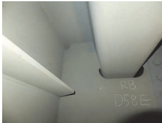
D58 diaphragm, east face. No cracks. Above this area, pavement cracks exist.
