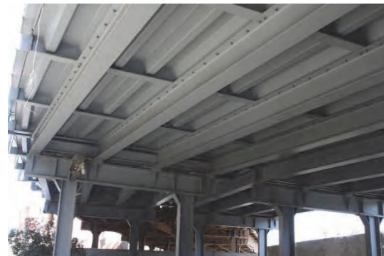
3. Panels of orthotropic steel deck were fabricated at the shops and transported to the site and assembled. One panel is about 8m long, if lateral rib spacing is 2m, and consists of 6 U-ribs. The U-rib directly above the longitudinal beam is not a U-rib but it consists of two inclined plates.
