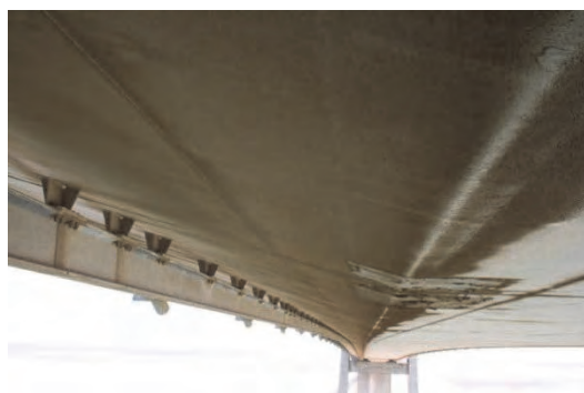
6. Sand covered bottom plate
