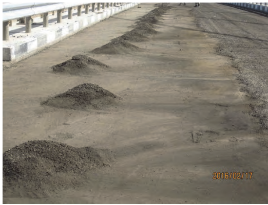
1. Surface after removal of pavement.
