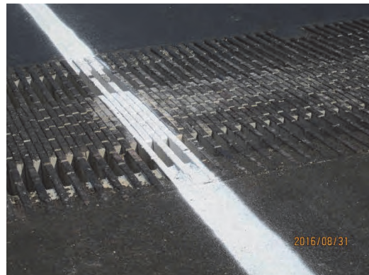
The pavement around expansion joint of East end.
