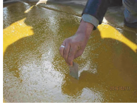
6. Measurement of thickness; A little too thick, so it will be reduced more totargeted 0.05mm on actual stage.
