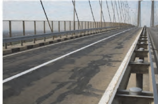
4. On the south lane, the pavement crack over R4 U-rib is not formed.
