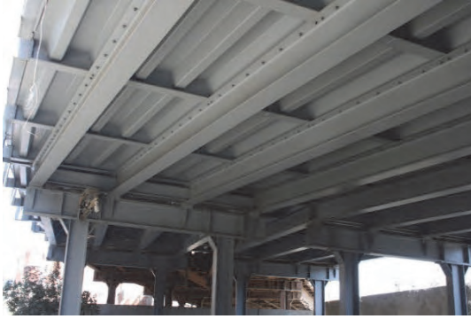
5. Panels of orthotropic steel deck were fabricated at the shops and transported to the site and assembled. One panel is about 8m long, if lateral rib spacing is 2m, and consists of 6 U-ribs. The U-rib directly above the longitudinal beam is not a U-rib but it consists of two inclined plates. The south side lane consists of two panels and the north side lane also consists of two panels.
