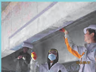
Undercoating of Epoxy adhesive
