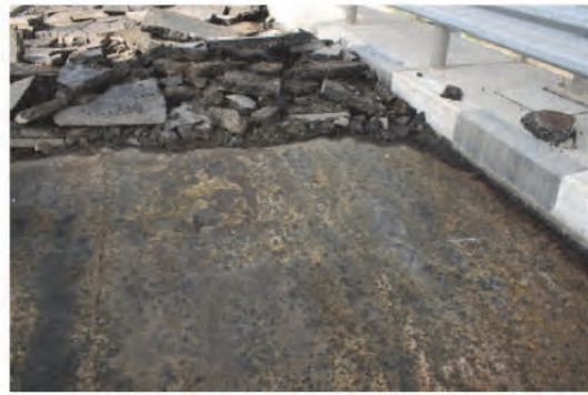
8. Corroded area near the west tower. This may be worst corroded.
