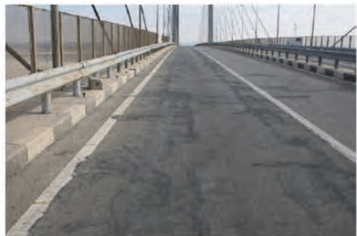
5. Near the bridge center, a crack line over R4 is not formed.
