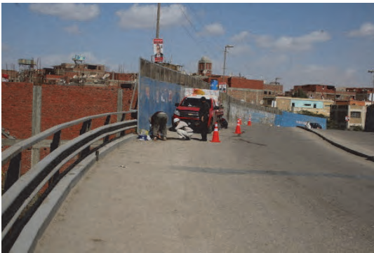
13. On the bridge deck, the pavement was investigated.
