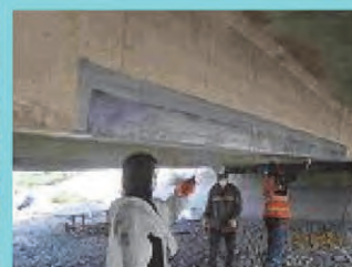
Final coating of Epoxy adhesive
