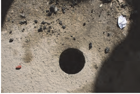
17. Drilled hole for core sampling.
