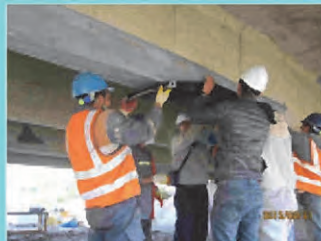
Setting of CF (Carbon-fiber)
