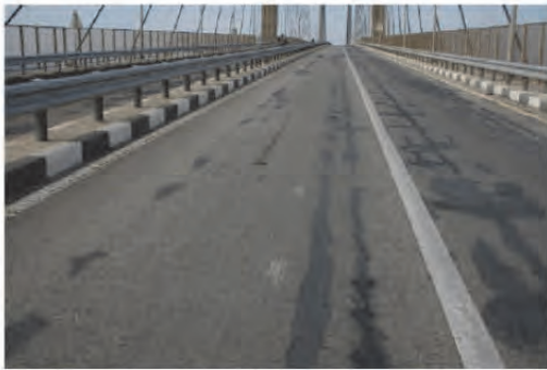
1. East side of the bridge and north lanes. Looking towards West on Overtaking Lane. Line repairs of pavements are visible.
