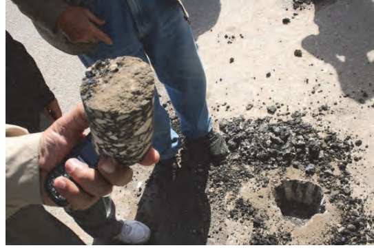
18. Drilled core. The pavement is healthy.
