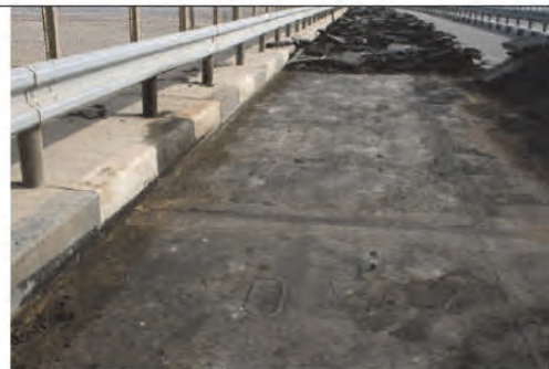
6. Near the tower, pavement materials were removed and the starving horse is visible. A temporary hand hole is between R4 and R5.
