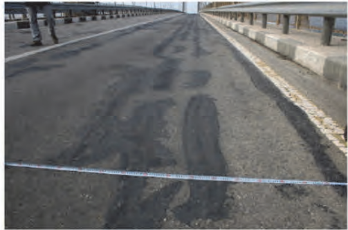
3. In this area, a repair line near the right white line, which is at the center of R4, is visible. But over this line, tires do not run so often and the reason of the crack formation is unclear.
