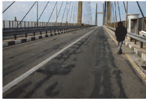
2. Driving Lane and 5 lines of pavement repair are visible. These lines correspond to the center of the U-ribs or the center of two adjacent U-ribs. This will be explained in detail, later.
