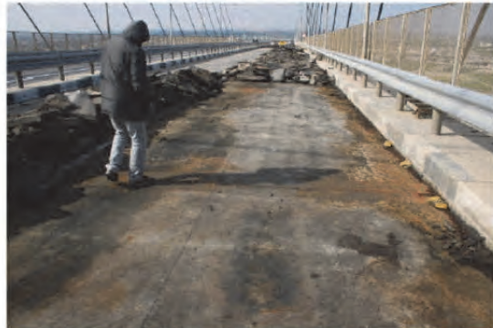
10. The corroded areas are on both sides which are below the cracked pavement areas. The center area is healthier.
