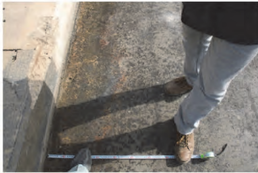
7. The welding line of R4 U-rib below the steel deck, which is 64cm apart from the curb is visible on the left of the brown shoes.
