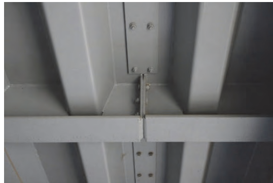
8. Connection of adjacent panel. U-rib details are quite fine.
