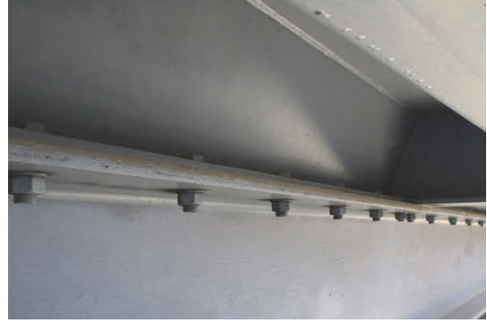
12. Inclined plate above the longitudinal beam. The structure is well-designed. No sign of fatigue cracks were found.
