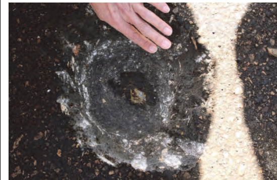
4. Condition of pavement was quite good and no rust was observed on the deck surface. The yellow color shows the Zinc Chromate. Hexavalent(+6) Chrome is toxic but Trivalent(+3) Chrome is not.
