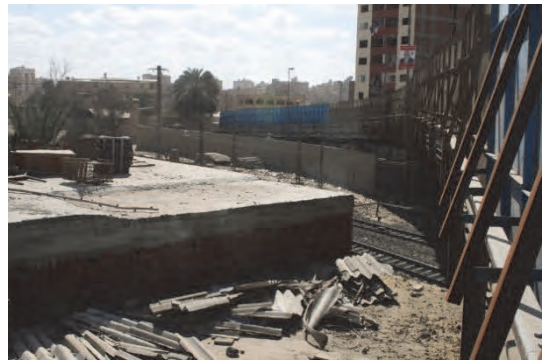
2. The Maasara Bridge, this bridge was constructed hastily, that was the reason why the orthotropic steel deck was adopted. Subway tracks can be seen on the left, North side.
