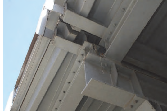
6. The open trapezoidal shape directly above the longitudinal beam shows the U-rib which consists of two inclined steel plates.
