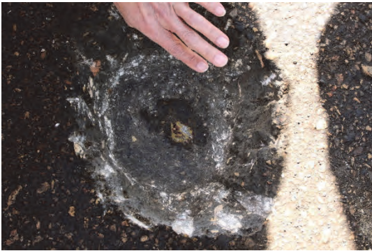
15. Condition of pavement was quite good and no rust was observed on the deck surface. The yellow color shows the Zinc Chromate. Hexavalent(+6) Chrome is toxic but Trivalent(+3) Chrome is not.
