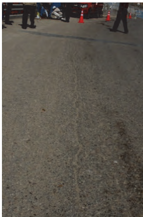
9. Cracks on the pavement. These cracks seem to correspond to the position of two panel connection, because two panels can move independently to some extent.
