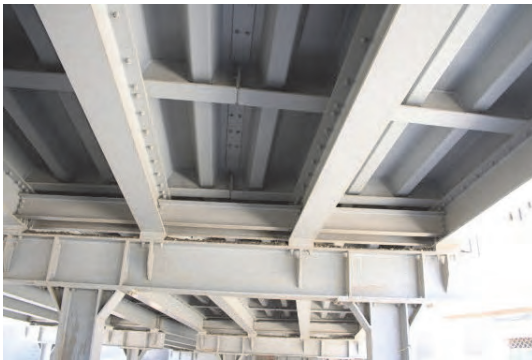
7. Two panels are connected at the center of south lane.
