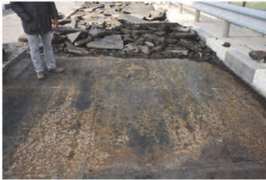
9. Corrosion near the west tower and on the North Lane.
