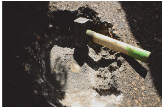
16. Size of the hole on the deck
