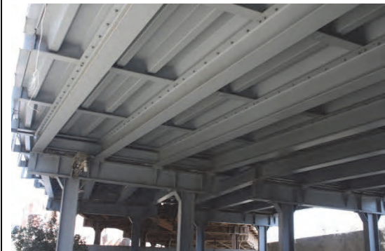
3. Panels of orthotropic steel deck were fabricated at the shops and transported to the site and assembled. One panel is about 8m long, if lateral rib spacing is 2m, and consists of 6 U-ribs. The U-rib directly above the longitudinal beam is not a U-rib but it consists of two inclined plates.
