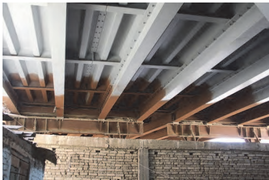
19. In 1994, both sides of the bridge was painted by Zinc Rich Paint. But Subway Company refused to paint the center of the bridge. It is said that the weathering steel was adopted for this bridge. Then it was not needed to paint.
