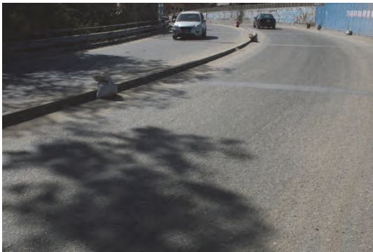
1. The Maasara Bridge over Subway. On the right is the South Lane.
