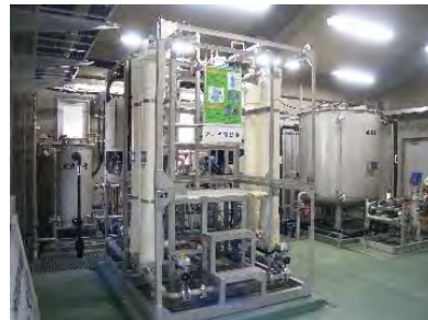
Membrane filtration facilities, Water supply system for Kuroda area in Kyoto city, Waterworks Bureau, City of Kyoto http://www.city.kyoto.lg.jp/suido/page/0000160981.html
