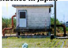
Lifting phenomena at pumping facility
