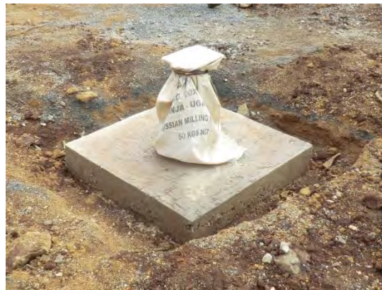
Protected borehole after drilling
