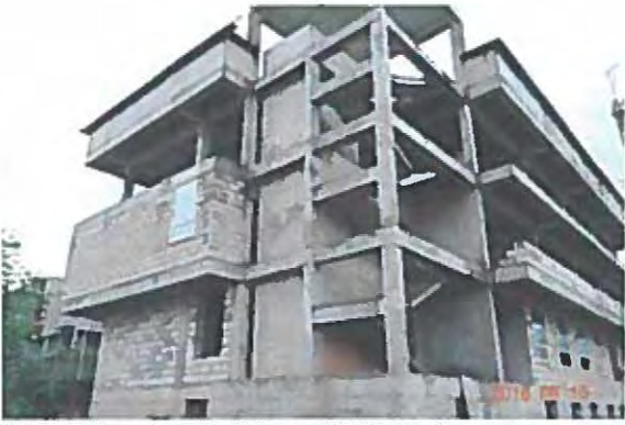
New Laboratory Building of IVM (under construction)
