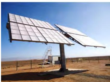
Figure 16 : The Tracker Position (Left: Tracking in Daytime, Right: Standby at Night)
