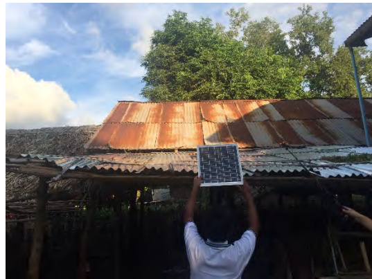
Figure 2.12: Install solar panel at purchaser's house
