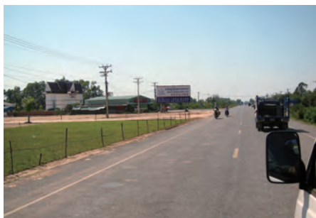
Road condition of NR 5
