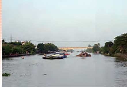
Electric cable above Chi Gao Canal
