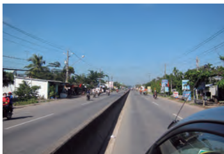
Road condition of Vietnam Side
