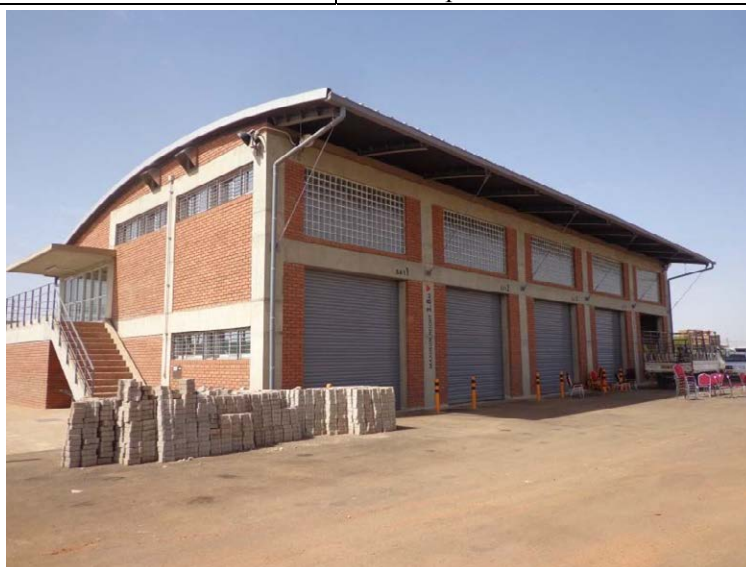
Fig. 1-3 Picture of Central Workshop (for Vehicle Maintenance) Constructed by Related Grant Aid Project
