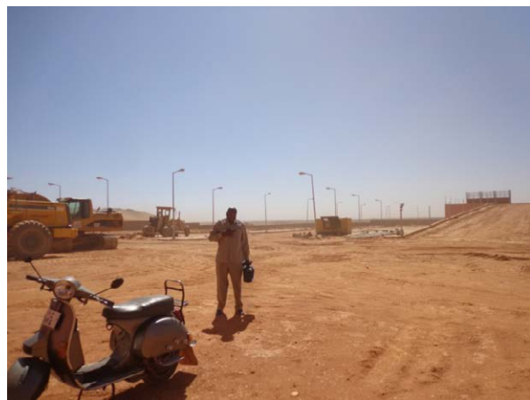
Umbadda transfer station construction by Khartoum state
