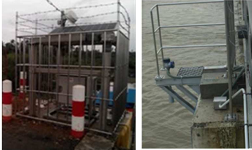
Photo 1 Installed automatic tide gauge
