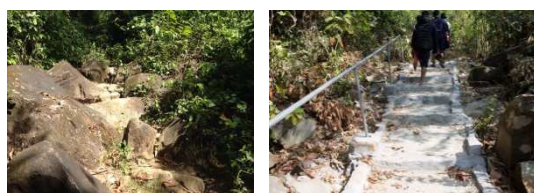
Photo 5 Evacuation route constructed by Community Infrastructure Support Project (Before: Left, After: Right)
