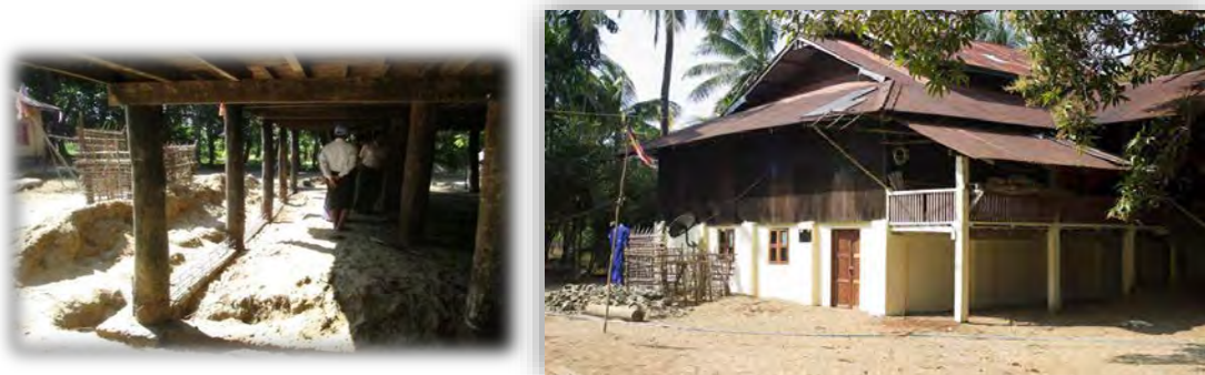
Figure 4.7 Monastery Under Construction (Left) : Monastery After Retrofitting (Right)
