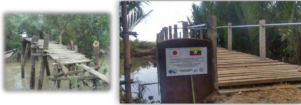
Figure 4.6 Bridge before reconstruction and after reconstruction
