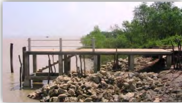
Figure 4.3 Jetty after reconstruction
