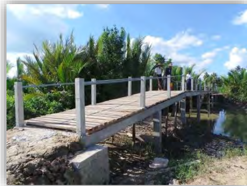
Bridge under the construction
