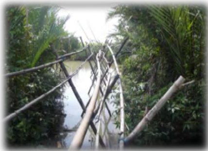
Figure 4.4 A simple bridge connecting paddy field to residential area
