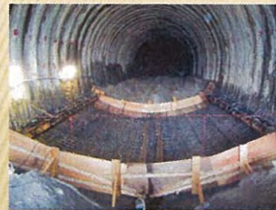
Invert under construction
