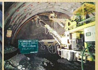
Erecting Steel Supports
