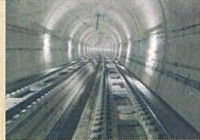
Tunnel and Slab Track
