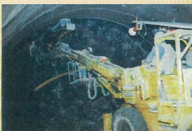
Erecting Steel Support
