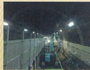
Repairing work of the invert
