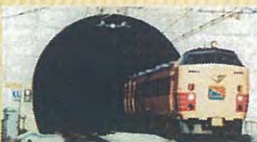
Seikan Undersea Tunnel
