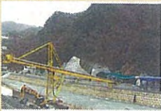
Photo 1 Belt conveyor outside the tunnel
