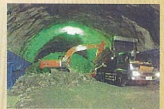
Temporary storage of excavated muck in the tunnel
