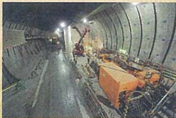
1,000m-class ultra-long pilot boring
