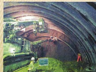
Erecting Steel Supports
