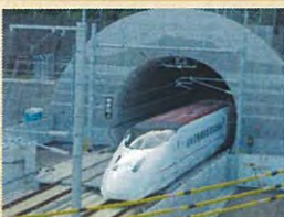
Kyushu Shinkansen Tunnel
