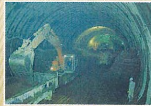
Mucking in the tunnel
