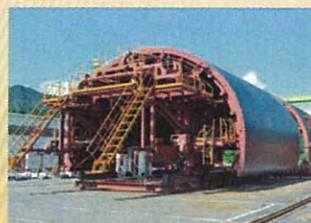
Form for Tunnel Lining
