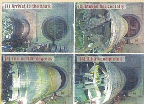
U-turn Process of the Shield Machine
