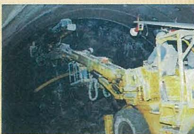
Erecting Steel Support
