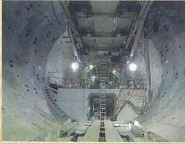
Shield Tunnel under Construction with Ceiling Crane & Escape Passage
