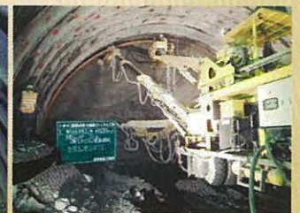
Erecting Steel Supports
