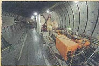
1,000m-class ultra-long pilot boring
