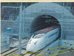
Kyushu Shinkansen Tunnel
