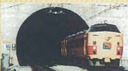
Seikan Undersea Tunnel
