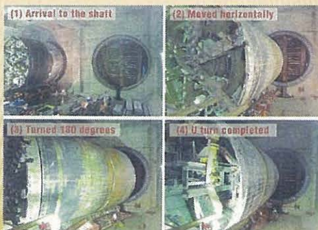
U-turn Process of the Shield Machine
