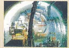
CRD Method for Settlement Measure
