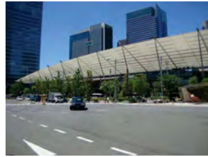
Tokyo Station Yaesu side(Grandroof)
