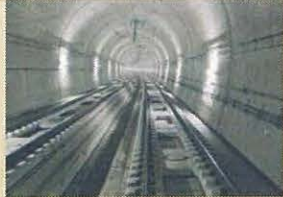
Tunnel and Slab Track
