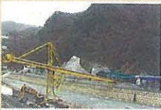
Photo 1 Belt conveyor outside the tunnel
