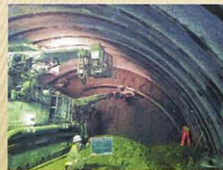
Erecting Steel Supports
