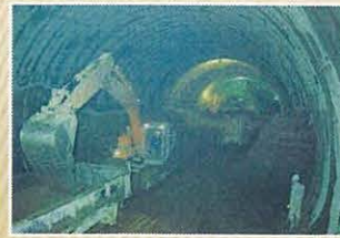
Mucking in the tunnel
