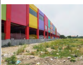
4. View of the Site
