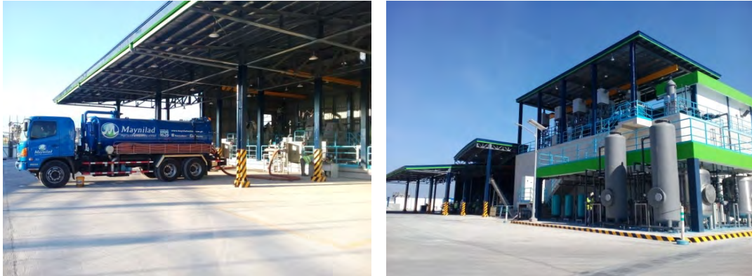
Figure 3.1.4 South Septage Treatment Plant
