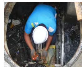
Figure 3.3.2 Cleaning Work in Manhole
