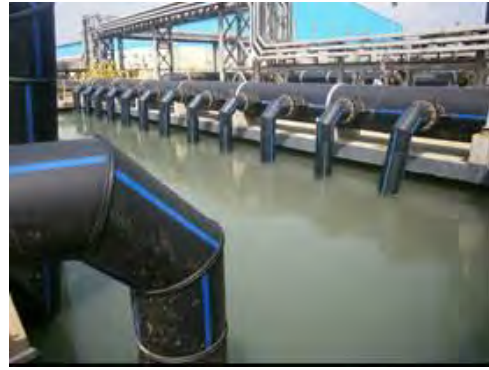
Picture A3.11.1 Up-flow filter in the Nemmeli DSP
