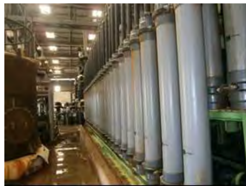
Picture A3.11.2 UF racks in the Nemmeli DSP
