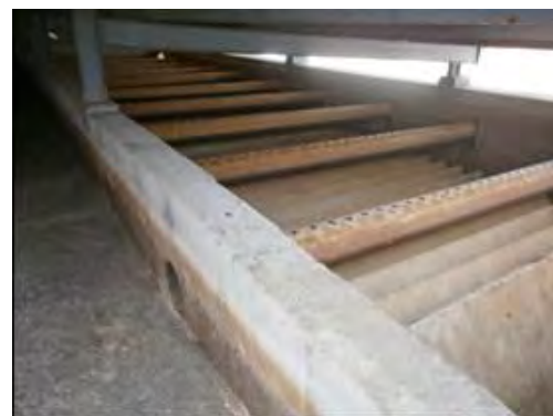
Picture A3.11.6 Gravity Settler in the Minjur DSP
