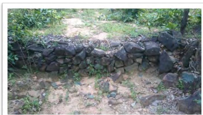
JFM activity - Loose Boulder Check Dam ( LBCD) in Arjunabila VSS, Keonjhar District
