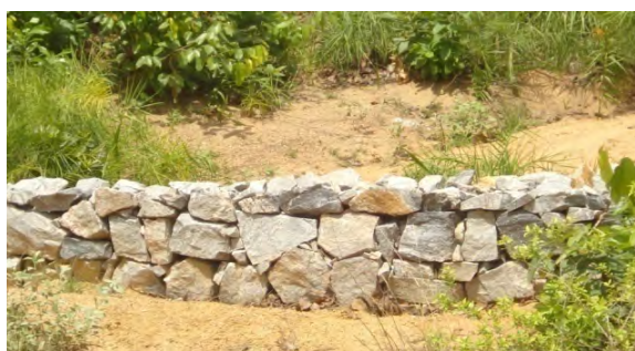
Loose Boulder Check Dam ( LBCD) in Arjunbila VSS, Keonjhar District
