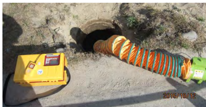
Figure 3-7: Detecting poisonous gas inside the joint box
