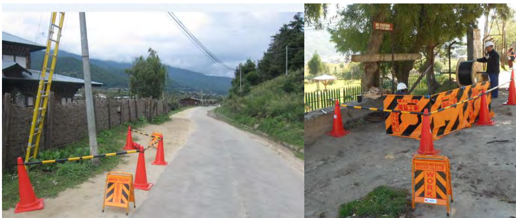
Figure 3-6: Safety measures on Aerial & Underground work
