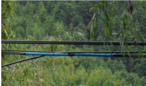
Figure 2-16: Cable passing through trees and bushes & CATV
