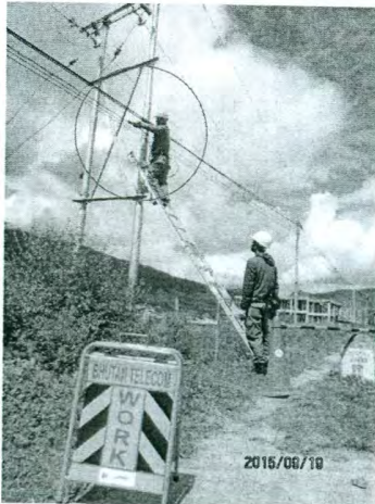
Protecting the fiber cable by using Protective sleeve from the electric leakage and
