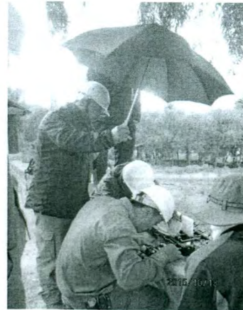
Protecting Splicing machine from rain and dust during Splicing of UG cable.
