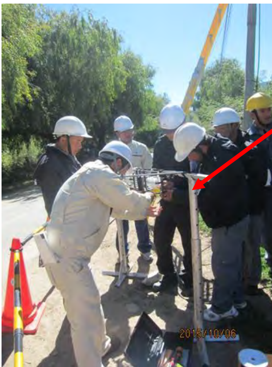
Phot 9 Scene of Optic Fiber Connection Work on Handmade Workbench
