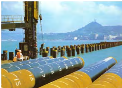
Figure 8.9-3 Heavy-duty Anticorrosion Lining (Urethane Elastomer)
