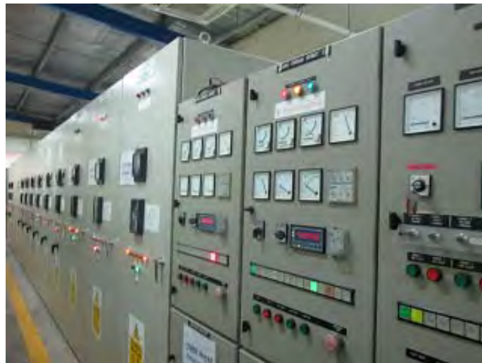
Figure 13.3-5 High-Voltage Incoming Panel in the Electrical Room in the Generator House
