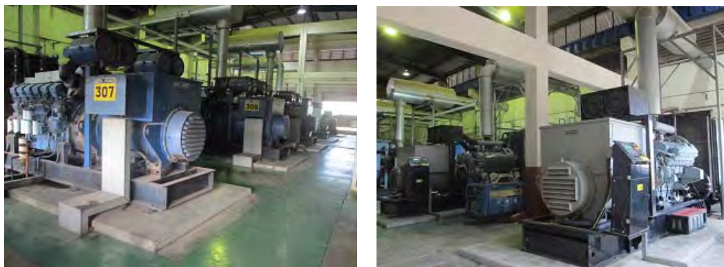
Figure 13.3-4 D-G Set (5 units) in Generator House
