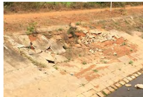
Picture 3.3.3 Damaged Canal Slope
