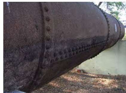
Picture 3.3.8 K1 Transmission Main (Riveted Steel) Installed in 1914
