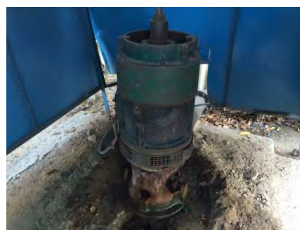
Picture 3.3.6 Deterioration of Well Pump in Poondi Wellfield
