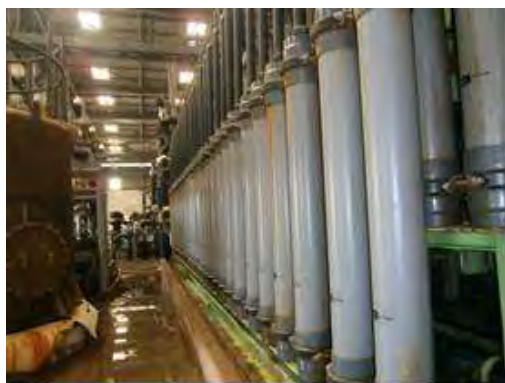
Picture 3.4.1 UF rack in the Nemmeli DSP
