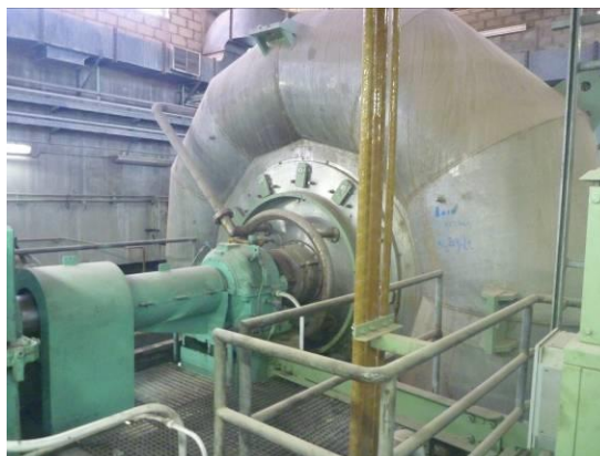
spillway small hydroelectric generator (Phase2)
