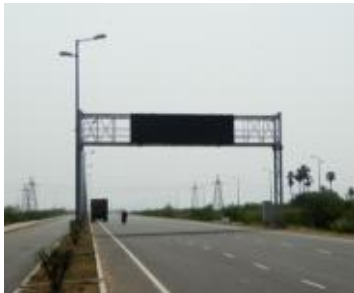
Figure 2.42 Variable Message Sign Board, Emergency Call Box, Meteorological Data System
