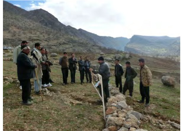
Joint work by three sectors (Forest and Rangeland, Community Development, Staff Training): Training on constructing terraces for Agroforestry and a check dam (December 2013, Gazestan village in Bazoft area)
