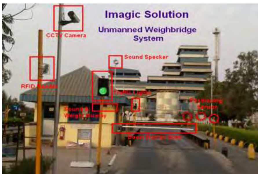
Figure 5.5.4 An Example of Automatic Weighbridge
