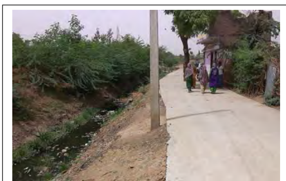
Status of canal near Swaroopganj
