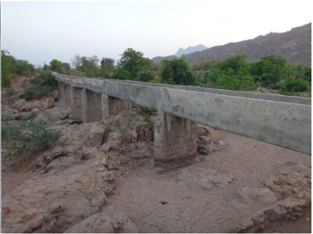
Aqueduct (flume to be replaced)
