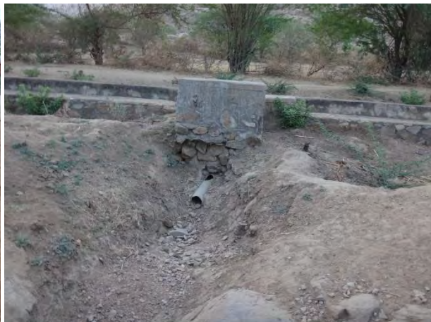
Outlet (to be rehabilitated)
