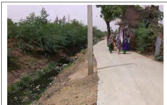
Status of canal near Swaroopganj
