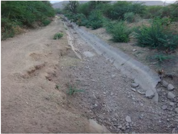
Main Canal (to be rehabilitated)
