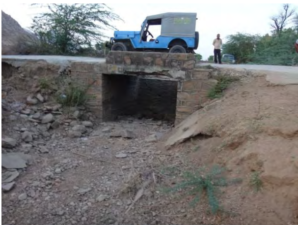
Fall with VRB (to be rehabilitated)
