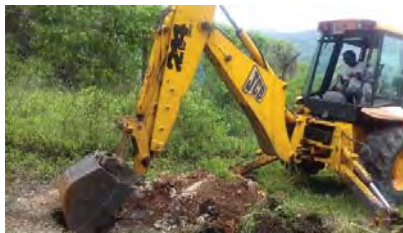
Figure 9 Picture of equipment used in digging of geological pit
