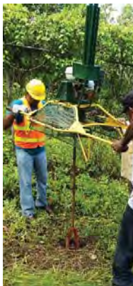
Figure 8 Picture showing initial boring of hole, Shotover, Portland
