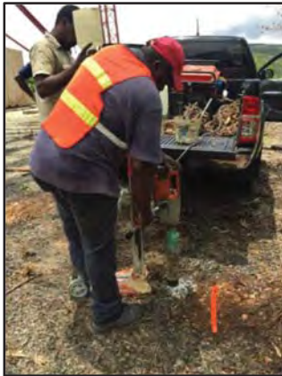
Figure 39 Picture showing use of coring machine at Winchester Site
