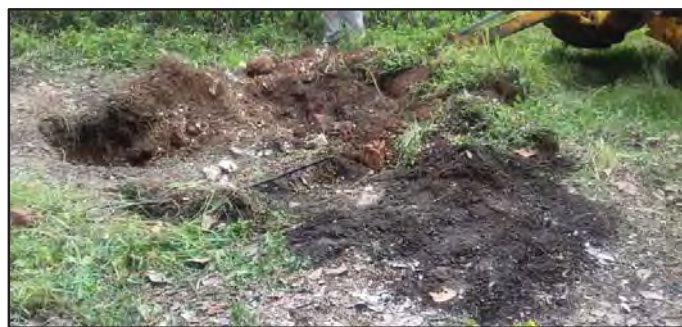
Figure 7 Picture showing unearthed soil at site
