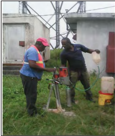
Figure 35. Picture showing use of coring machine at Cabbage Hill, St. Thomas
