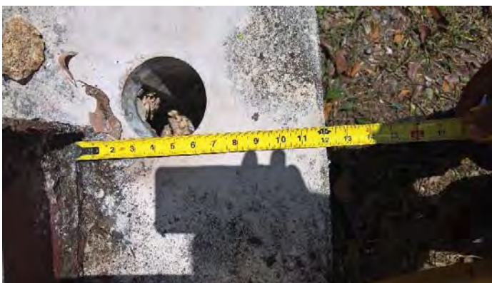
Figure 8. Picture showing location of second boring in southwestern corner of concrete base
