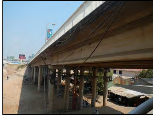
Communication cables attached to PC bridge (Optical fiber cables, etc)
