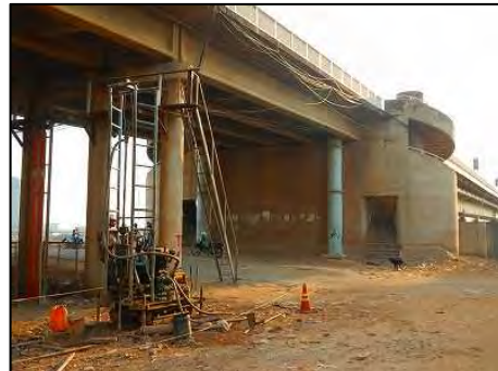
Photo 1-2-4 P8 pier boring (land)
