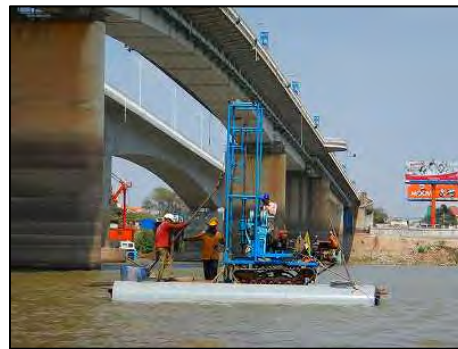
Photo 1-2-2 P3 pier boring (river)
