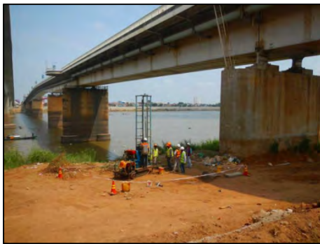
Photo 1-2-1 P2 pier boring (land)
