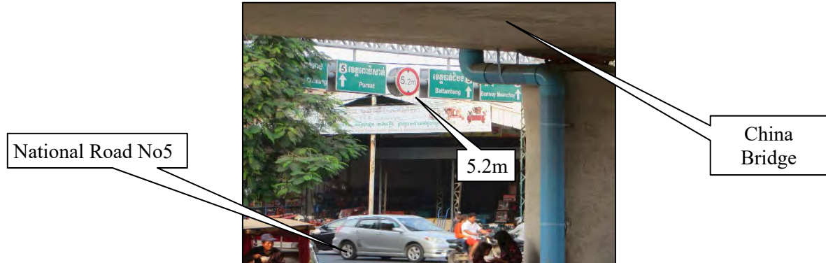
Photo 2-2-1 Vehicle Hight Restriction Sign
