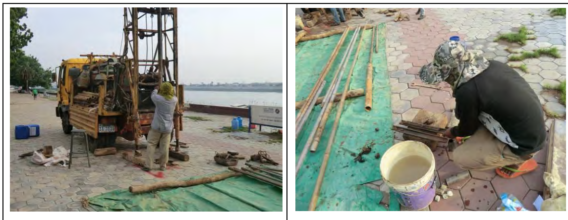
Photo R 1.3.3 Site Condition during the Boring Survey
