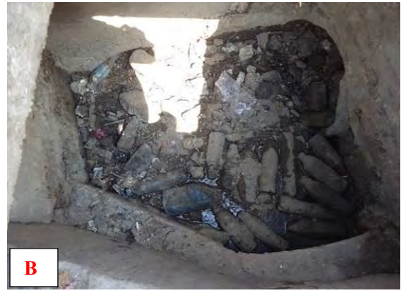
Fig. R 2.2.15 Clogging due to Deposition in Manhole (Left: St.528, Right: St.289)
