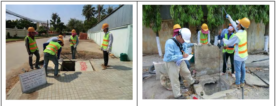
Photo R 1.3.2 Site Condition during the Manhole Survey
