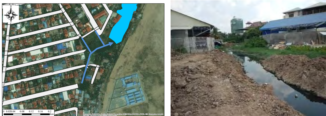
Fig. R 2.2.10 Open Channel Distribution Surrounding Tuol Kork2 (Left: Route of Channel, Right: Photo of Open Channel)
