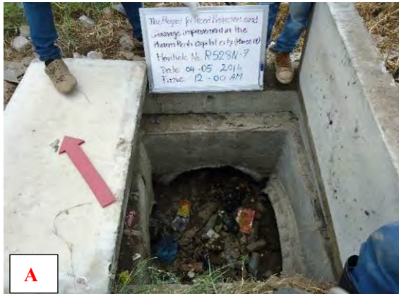
Fig. R 2.2.15 Clogging due to Deposition in Manhole (Left: St.528, Right: St.289)
