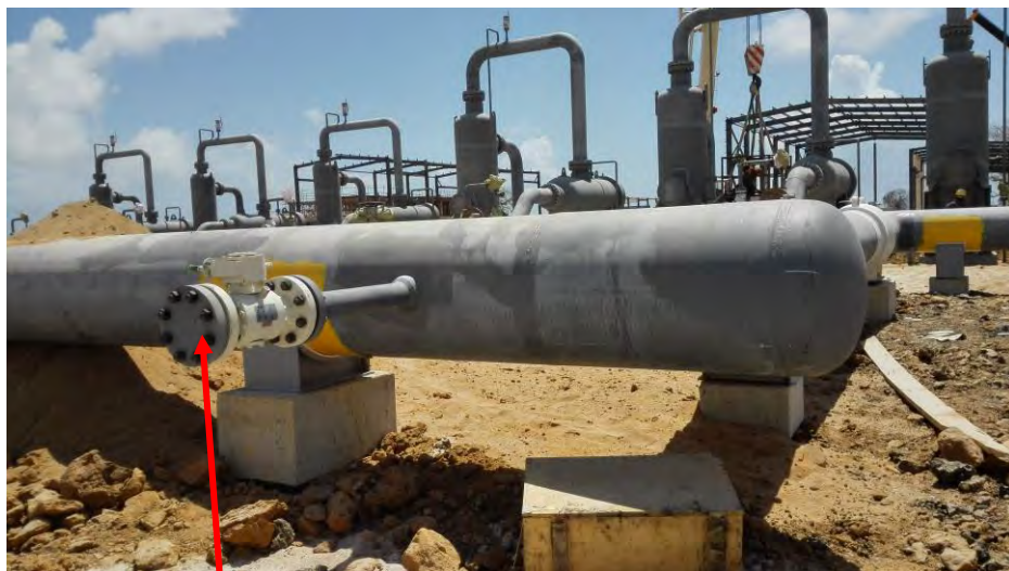
Typical tapping point at SomangaFungu. This point will supply natural gas to Kilwa Energy power plant and any other,
