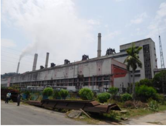
Obra 'A' Thermal Power Station
