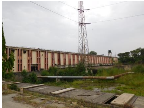
CWP Pump house (for Obra 'B')
