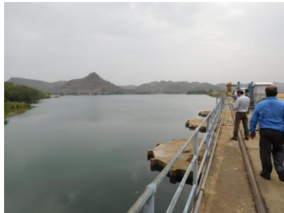
Obra Dam (Upstream)
