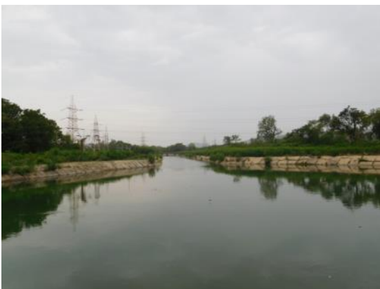
Water intake channel
