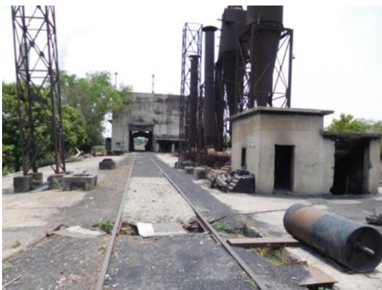
Coal unloading facilities
