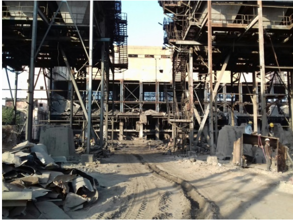
Boiler Building and ESP
