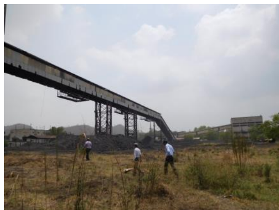
Coal storage yard (B)
