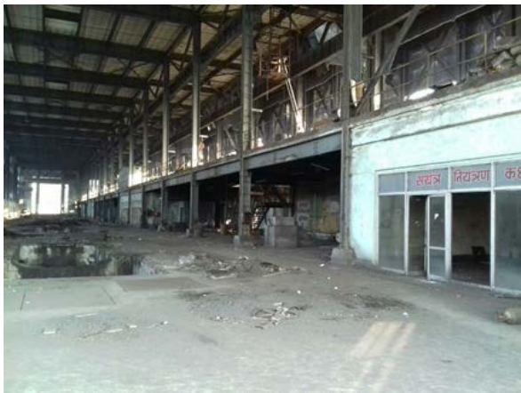
Turbine floor (HP Heater / CCR)
