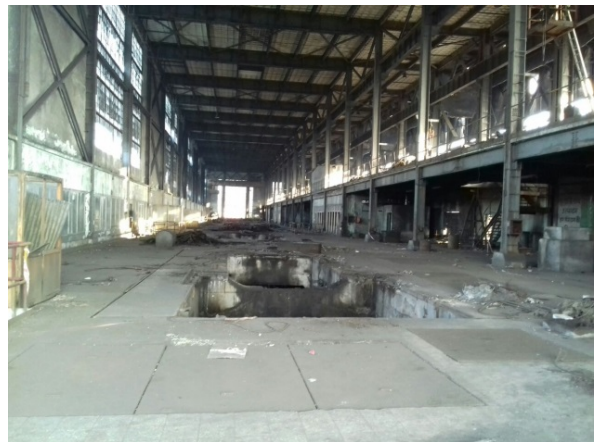
Turbine floor (TG base)
