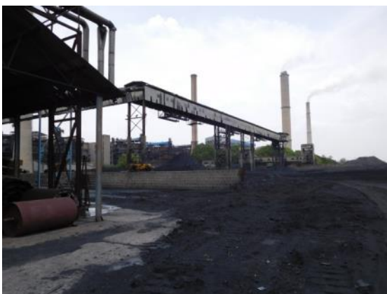
Coal storage yard (A)
