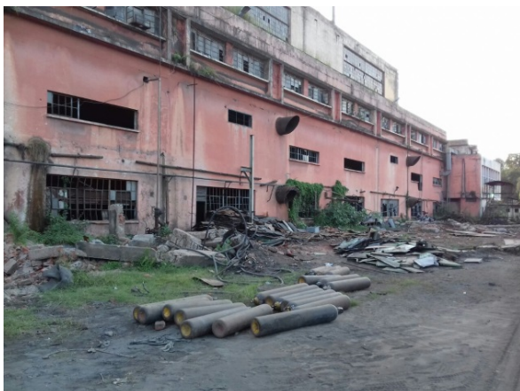
Turbine Building (Transformer)
