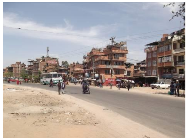
Remaining Houses in Right of Way (ROW)
