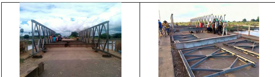
Photo 1-6-13 Construction of Bailey Bridge at Messalo I Bridge
