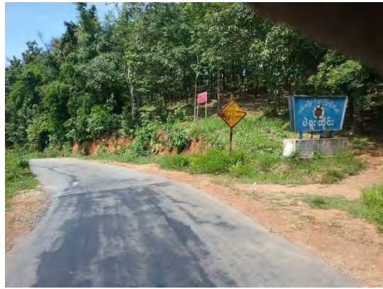
Existing Road Condition
