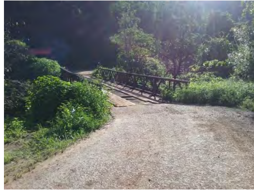
Existing Road and Bridge Condition
