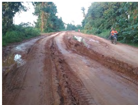
Existing Road Condition (Earth and Metal Road)
