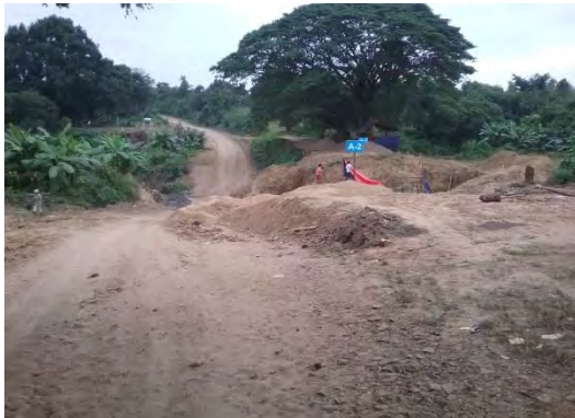
A Bridge Construction Area (MP 4/3) near Zebya Village
