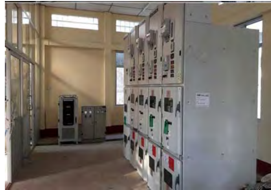
A Sample of 33/11 KV 5 MVA Sub-station
