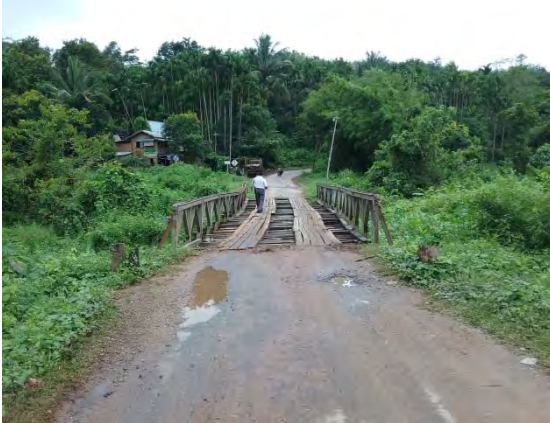
One of the bridges needed to be reconstructed
