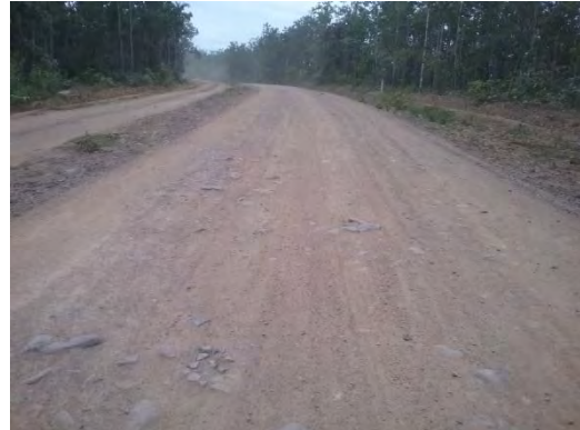
Existing Road Condition (Earth and Metal road)
