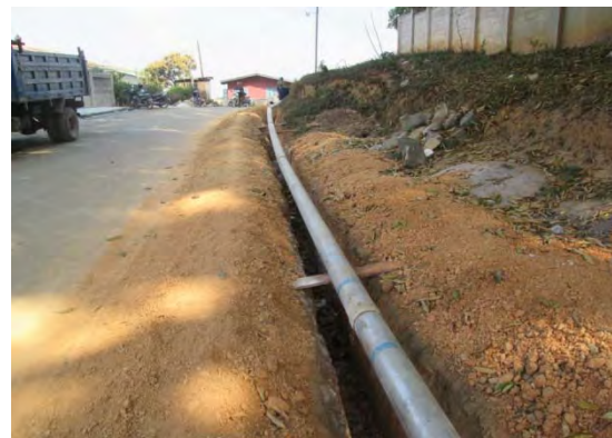
Pipe Line Installation
