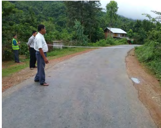
Existing Road Condition
