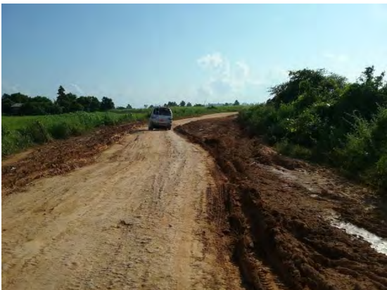
Existing Road Condition (Earth and Metal Road)
