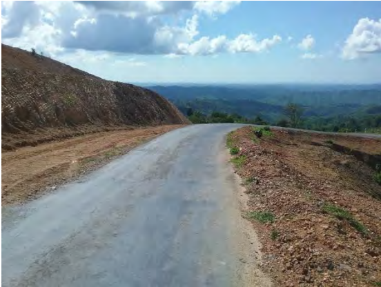
Existing Road Condition
