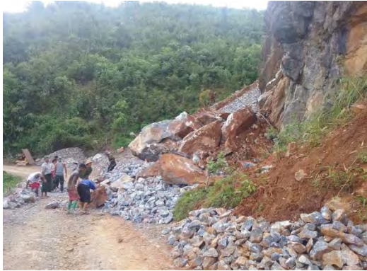
Embankment Widening by MOC Budget
