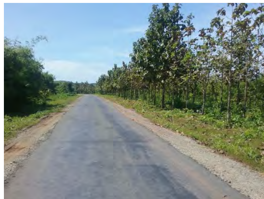
Existing Road Condition (12 feet Bituminous Road)
