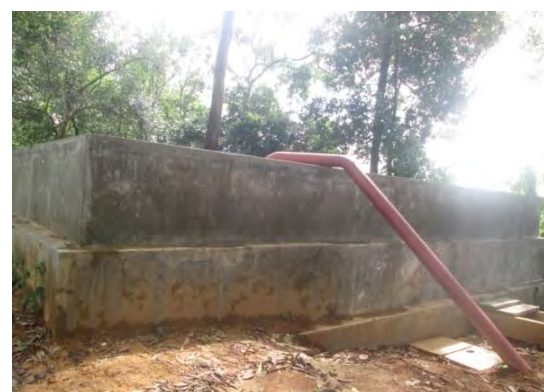
Clean Water Reservoir
