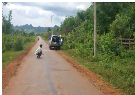
Existing Road Condition
