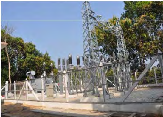
A Sample of 33/11 KV 5 MVA Sub-station
