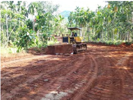
Embankment Widening by MOC State Budget.
