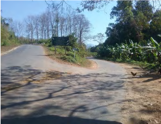
Starting Point of the project site (Bago Section)
