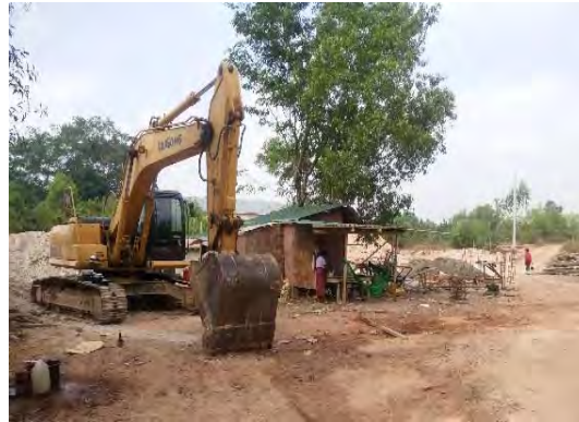
A Sample of Construction Stage
