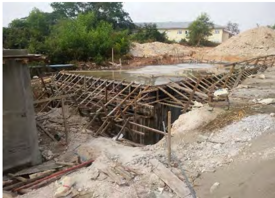
A Sample of Construction Stage
