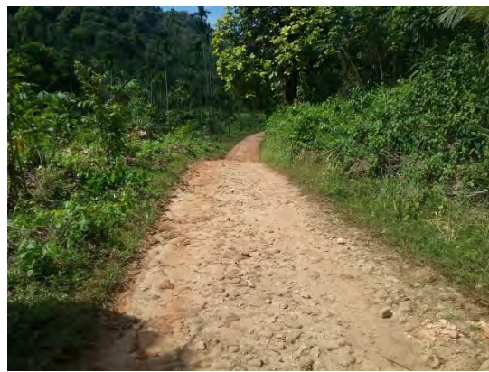
Some parts of Existing Road Condition (Earth and Metal Road)
