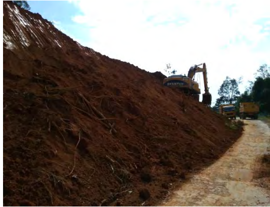
Embankment widening by MOC State Budget
