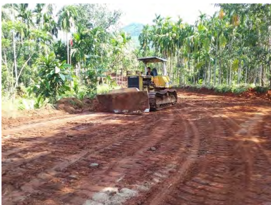
Embankment Widening by MOC State Budge.
