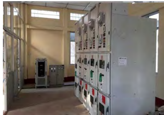
A Sample of 33/11 KV 5 MVA Sub-station
