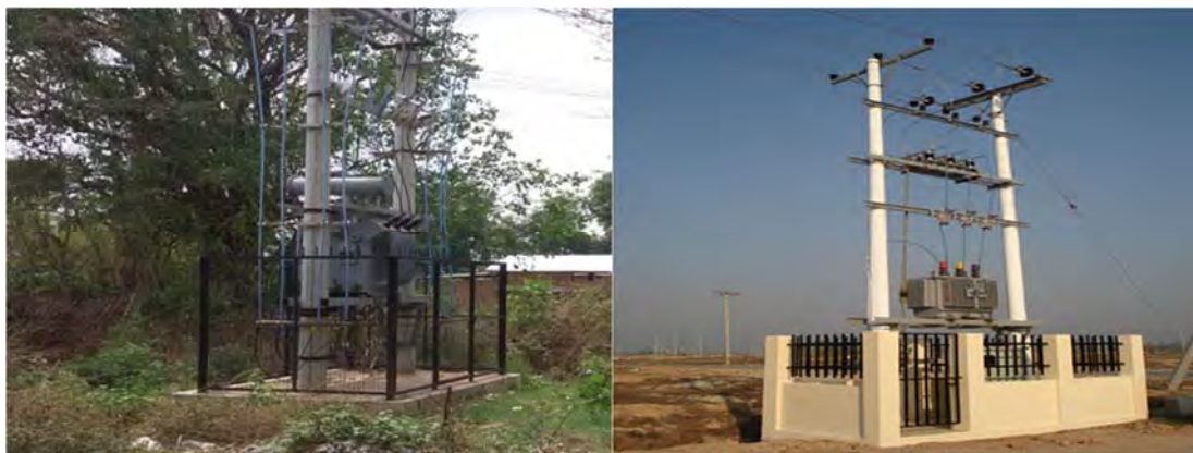
Samples of 11/0.4 KV distribution transformers
