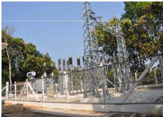
A Sample of 33/11 KV 5 MVA Sub-station
