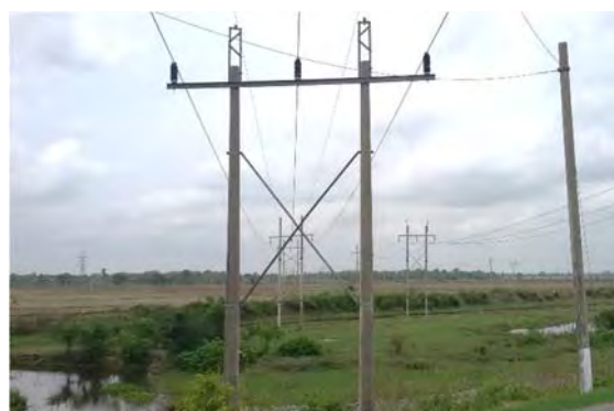
Samples of 66 KV Transmission Line
