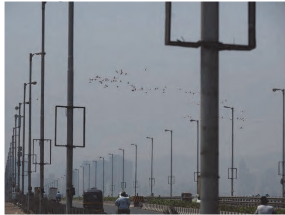
Flying over Airoli Bridge (the altitude is more than 20m)
